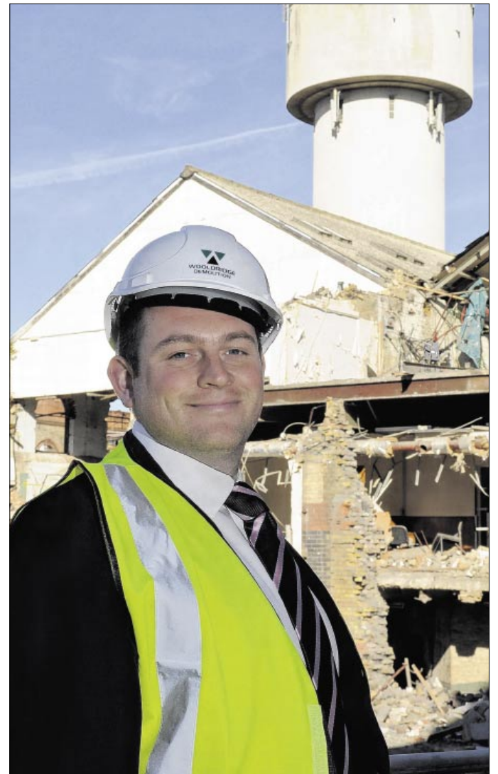
SUPERMARKET SWEEP: Essential Land Partner, Scott Hammond, at the site of the former paper mill in Milton Road
