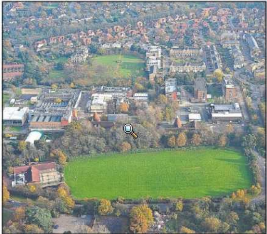
The old GlaxoSmithKline site in Beckenham could be redeveloped in a £150m scheme
